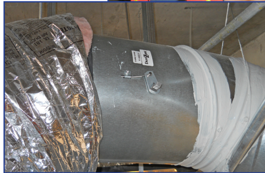
Installation of a Round Cable Operated Damper at the Marlin's Stadium.
