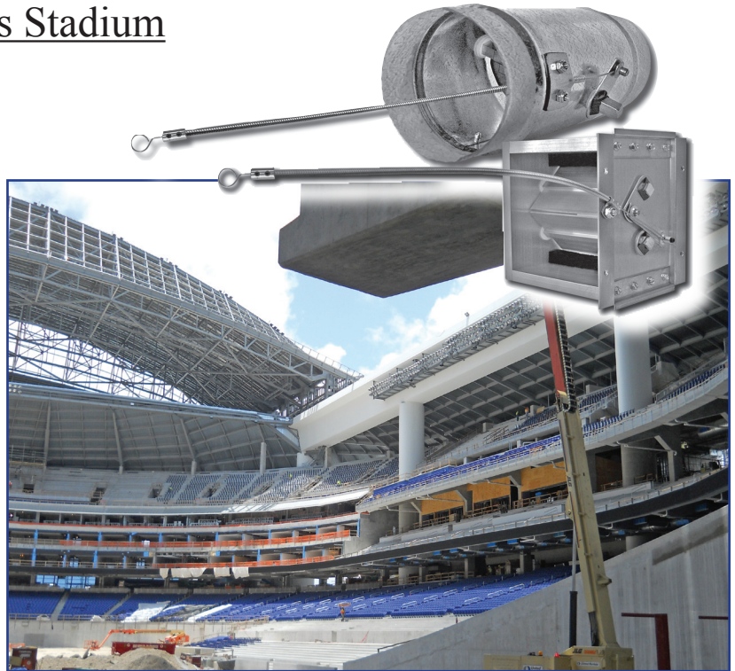
Marlin's Stadium Under Construction
