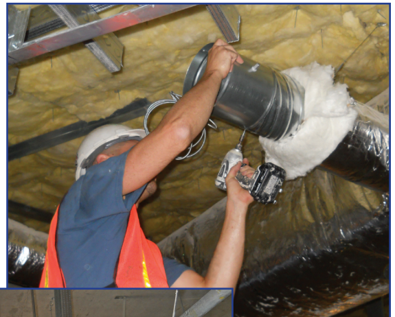
Installation of a Round Cable Operated Damper at the Marlin's Stadium.
